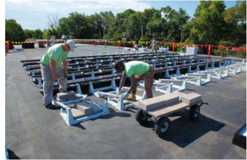
The result of their effort turned out to be a leap forward in solar rack systems. Called the DynoRaxx® Evolution, the 3-piece design requires no tools (can be installed with bare hands), is easy to transport, stronger and longer lasting than competitive products, and accommodates every PV solar panel on the market.
