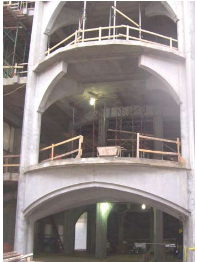
Fig. 5: View looking into the building, showing the gothic arches at the entryway as well as arched corbels featured in the rooms beyond and above
