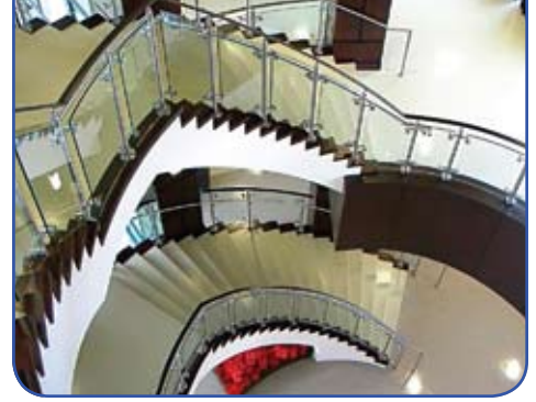
This dramatic view shows the finished stairway that was constructed with MFG CP concrete forms.
